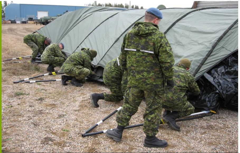
17 Wg pers setting up the COLPRO shelters during the camp build.
