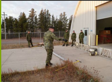
Cpl Keith Howard instructing the concrete screed
