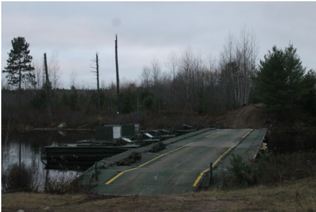
The finished bridge at Mount Batten.
