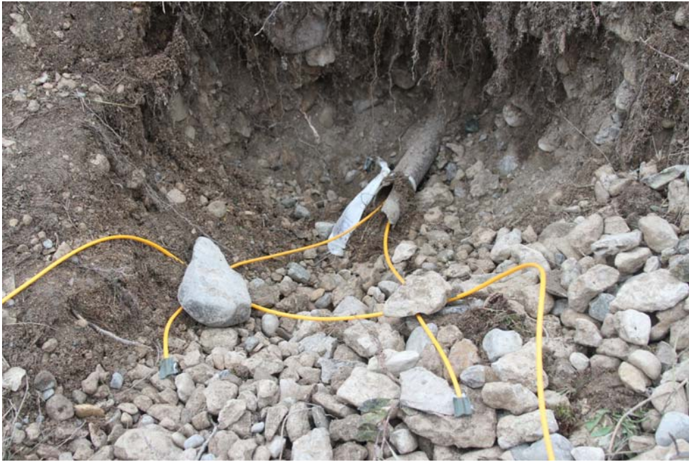
Pipe loaded with C4 charge to be burst into fragments
