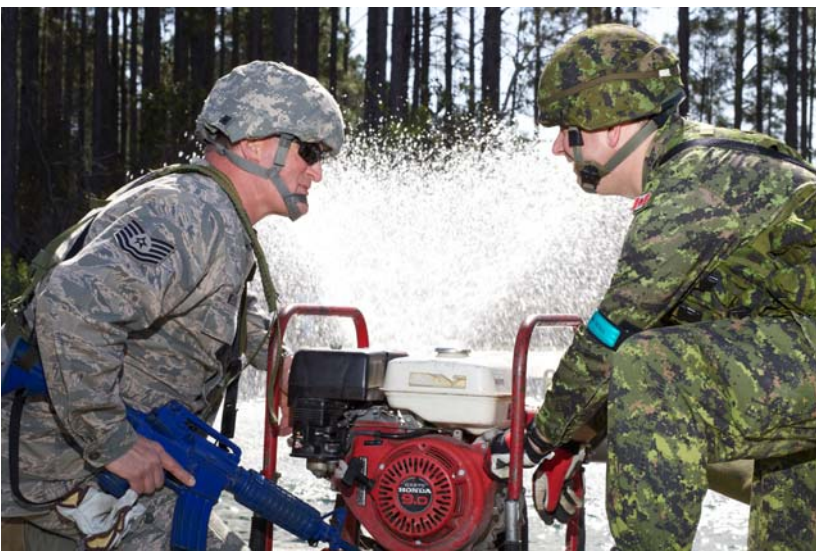
RCAF Cpl Donald Wray operates a portable water pump while preparing the water supply to the reverse osmosis water purification unit during the Silver Flag training exercise
