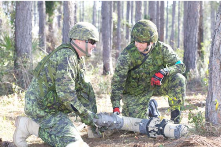
RCAF Sgt Joel Fitzgerald and RCAF Cpl Donald Wray connect piping for a water supply unit during the Silver Flag training exercise
