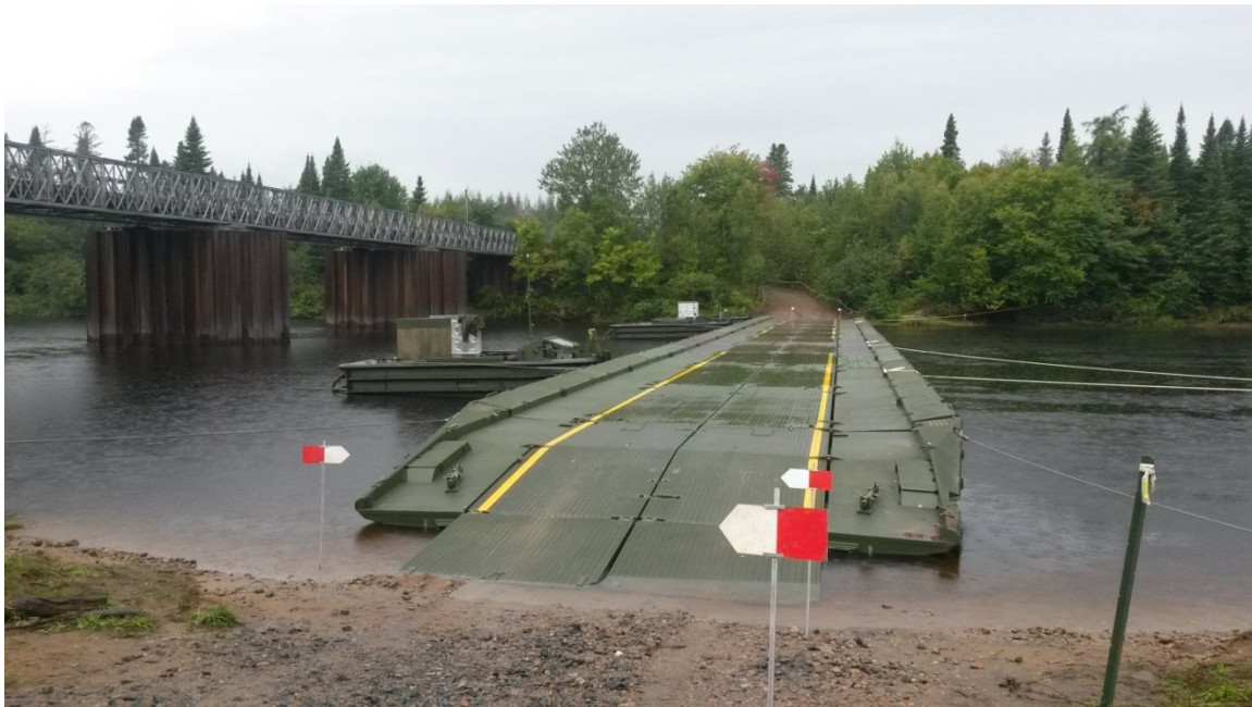
The 51 CER Field Squadron assembled a medium floating bridge that could support a vehicle of up to 70 tonnes over the Jacques-Cartier River.
