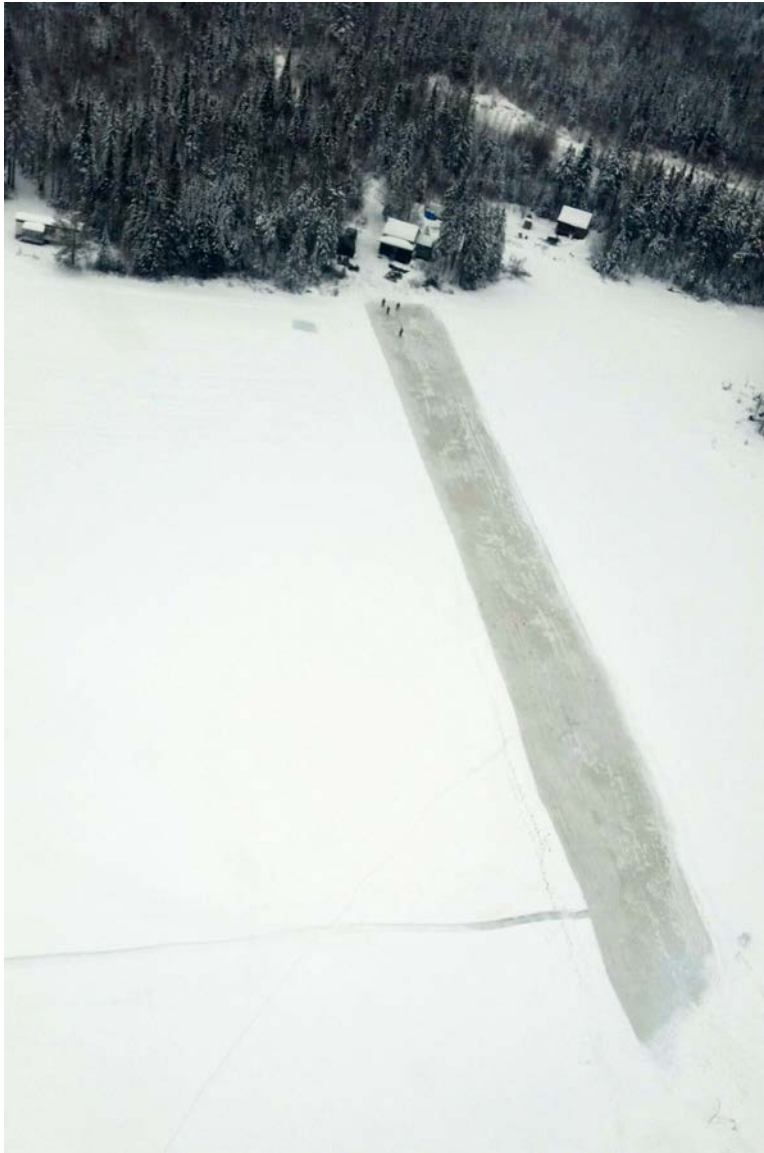
Aerial view of the ice bridge created by 35 CER engineers.
