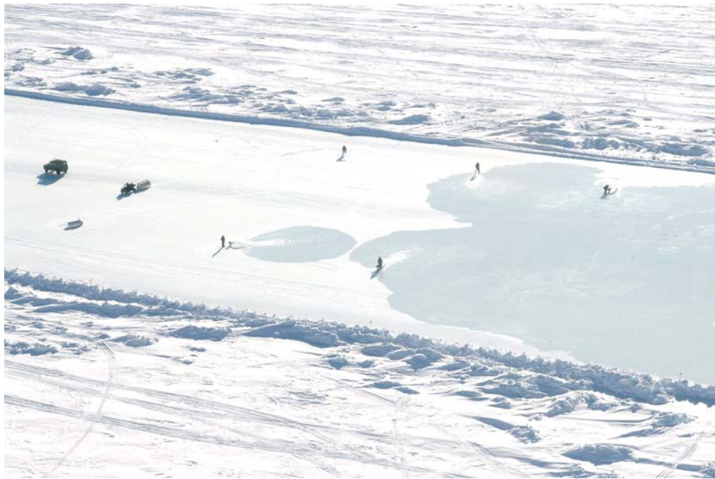
Members of 5 CER pump water onto the surface of the lake to create a runway strong enough to support a CC-130 Hercules.
