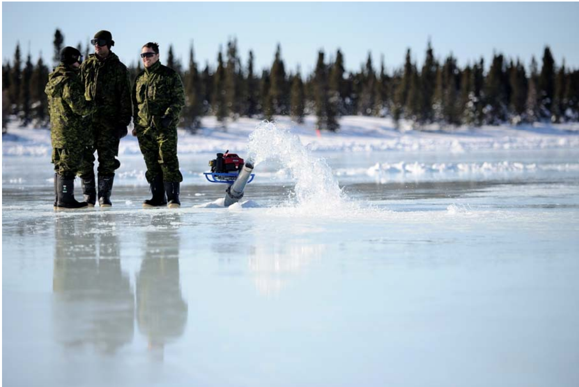
Members of 5 CER spray water to create a layer of ice on the ice runway.
