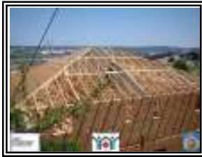
4 ESR Project nears completion St John, NB
