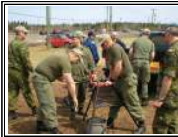
WCE Greenwood team constructs water cannon.
