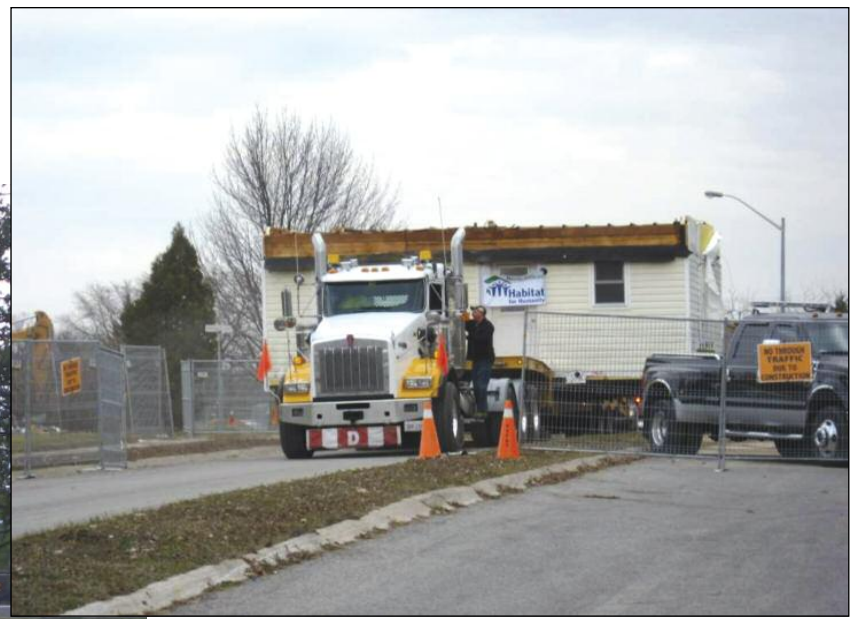
The ground floor of a housing unit is moved to a new site for a new family.
