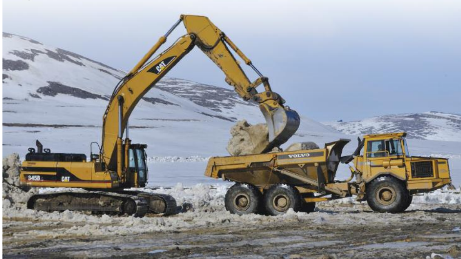
Soldiers from 4 ESR use heavy equipment to load snow into dump trucks to prevent chemical contaminants leaching from sources at the DEW line site into the Arctic ecosystem.
