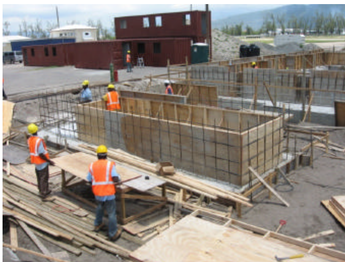
Alpha One Construction Site
