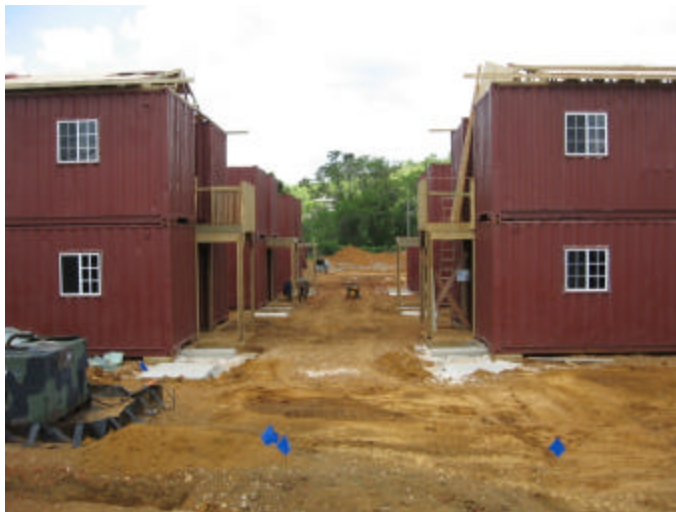
Camp Moneague Construction Site
