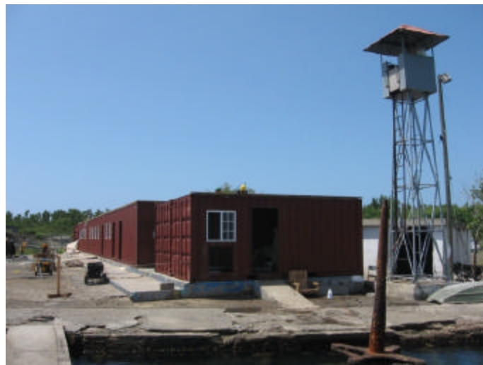
Coast Guard Construction Site
